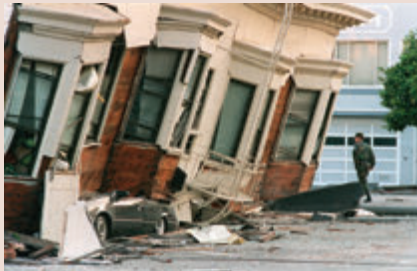
Collapsed apartment building in San Francisco, October 18, 1989, the day after the massive Loma Prieta earthquake
