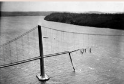
Collapse of the Tacoma Narrows Bridge
